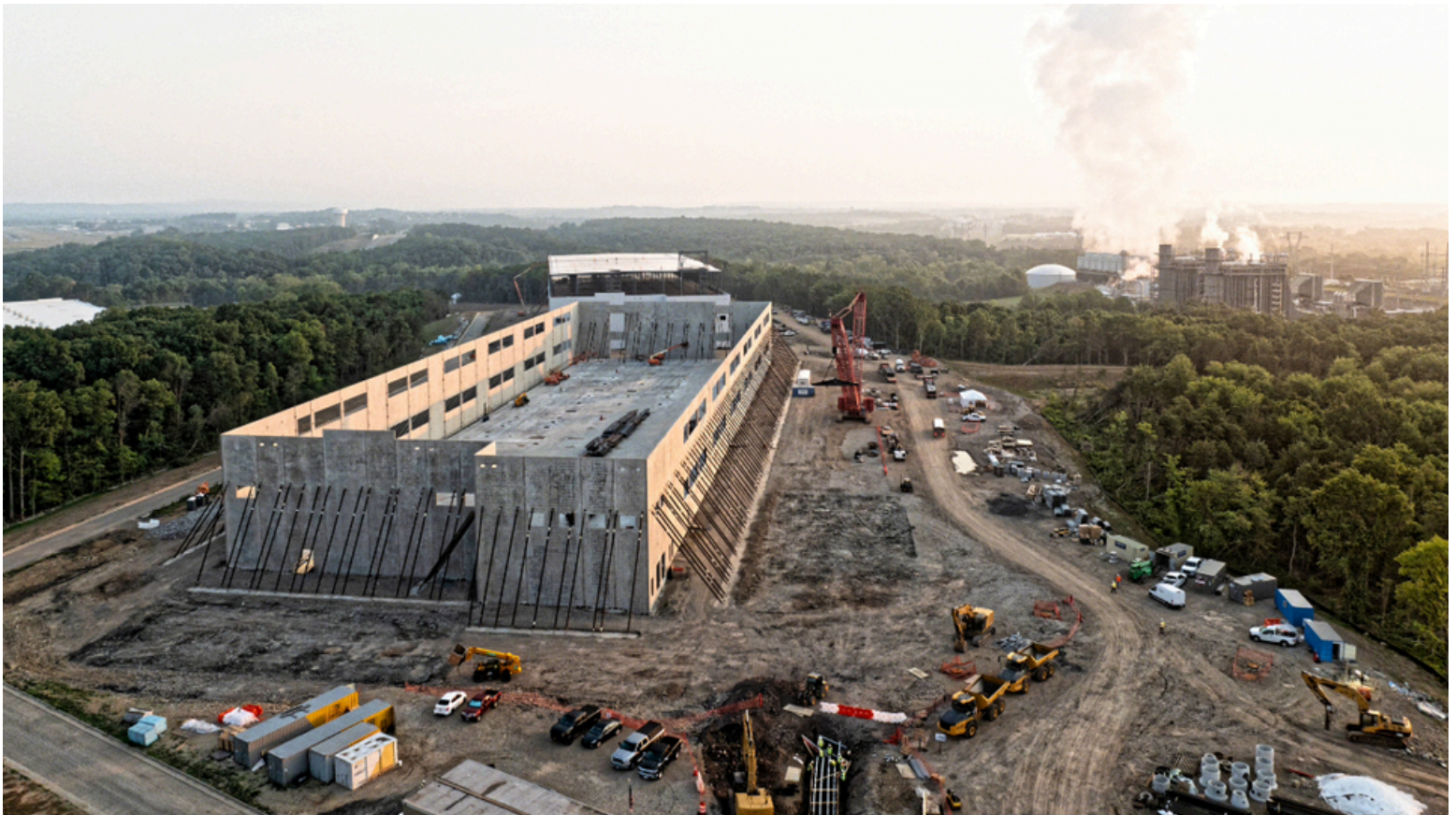
Data centers being built in Leesburg, VA (source: TechPolicy.press | credit: Gerville/2024)
